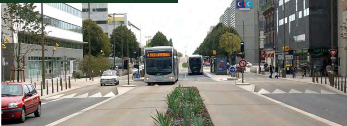
BusWay, Nantes Frankrike. Källa: COST TU0630 BHLS, Buses with High Level of Service, slutrapport
